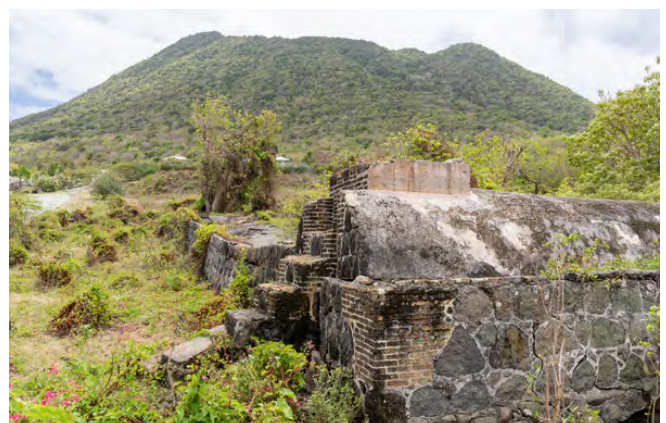
A gigantic cistern on the grounds of the former Knippenga plantation, St Eustatius. Collection of the Cultural Heritage Agency of the Netherlands, document no. BES-E-DSC08500. Photo: Robin Ammerlaan, RCE.
