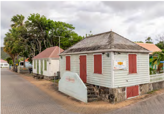
Paper Corner, a one-layer wooden house with shingles on the roof and wall and a stone foundation, Oranjestad, St Eustatius. Collection of the Cultural Heritage Agency of the Netherlands, BES-E-DSC09659. Photo: Robin Ammerlaan, RCE.
