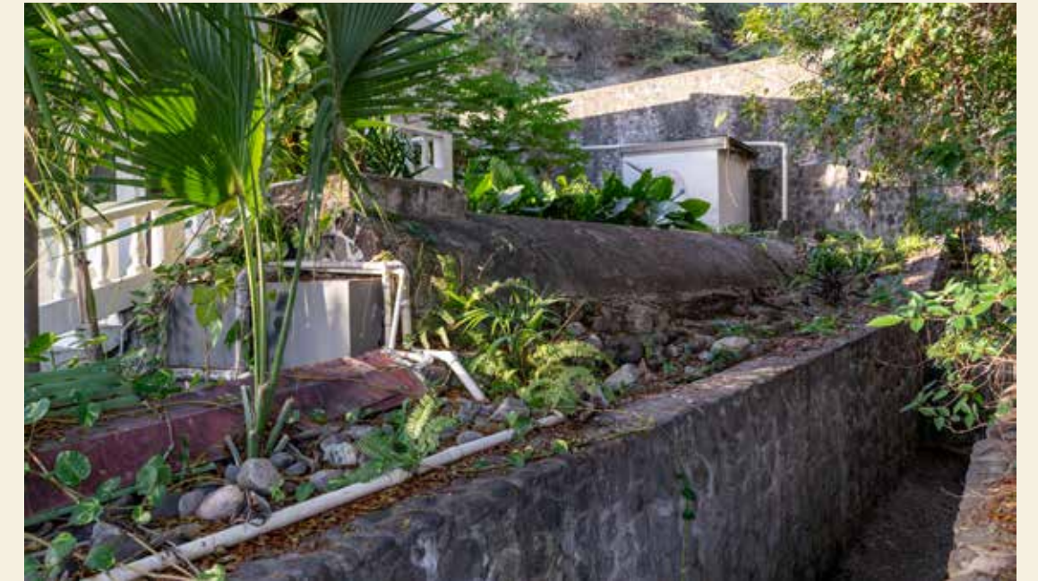
[Fig] One of Gin House’s largest cisterns. It has a capacity close to 60,000 liters.
