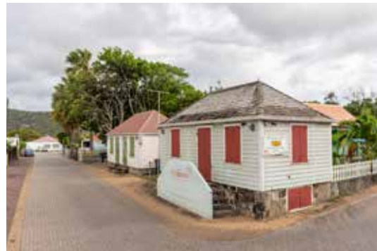
[Fig] The Government Guesthouse, stonework on the ground floor, wood above.
