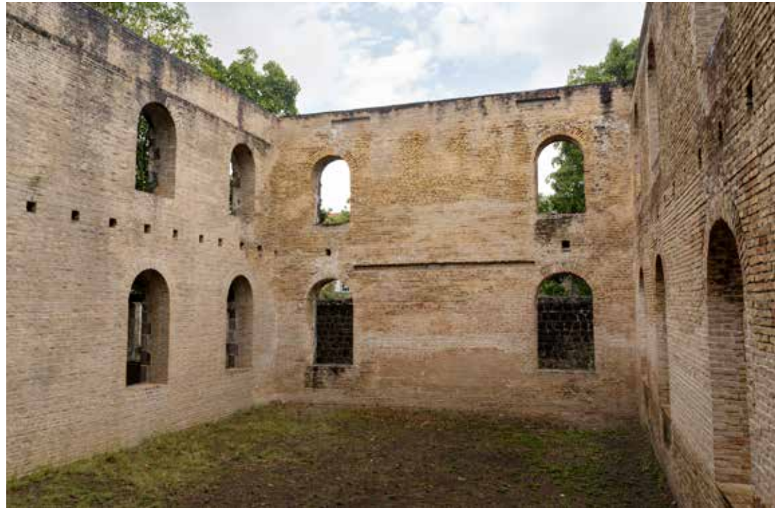
[Fig] Honen Dalim Synagogue after consolidation works.
