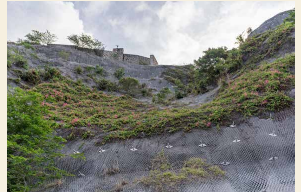
[Fig] Protective mesh around the cliff below Fort Oranje, designed to reduce erosion.
