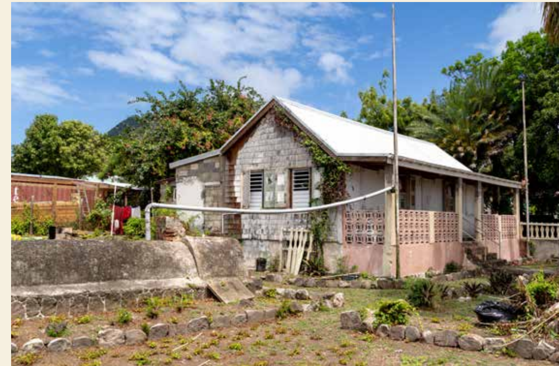
[Fig] Rainwater collected from a roof into a traditional cistern at a house in Oranjestad.
