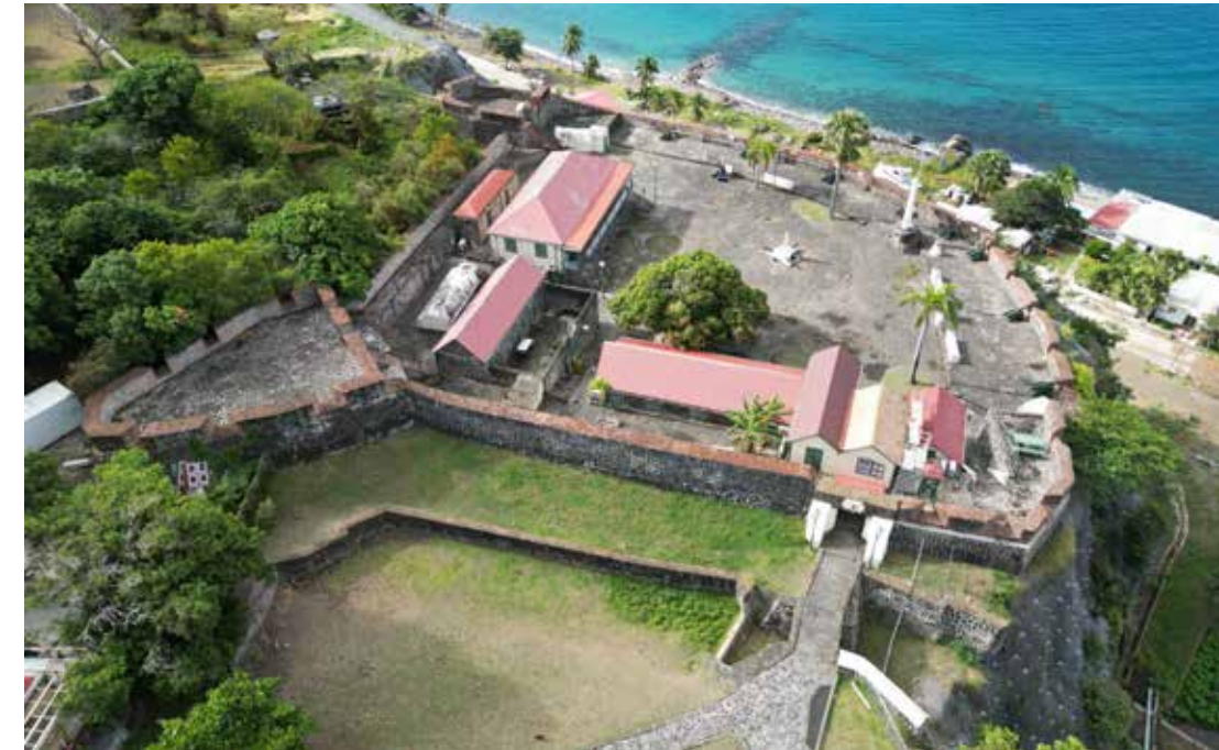
[Fig] Fort Oranje, on the edge of a steep cliff, is accessed by a bridge and gate. (photo: Michael Bacon, Alite b.v.)
