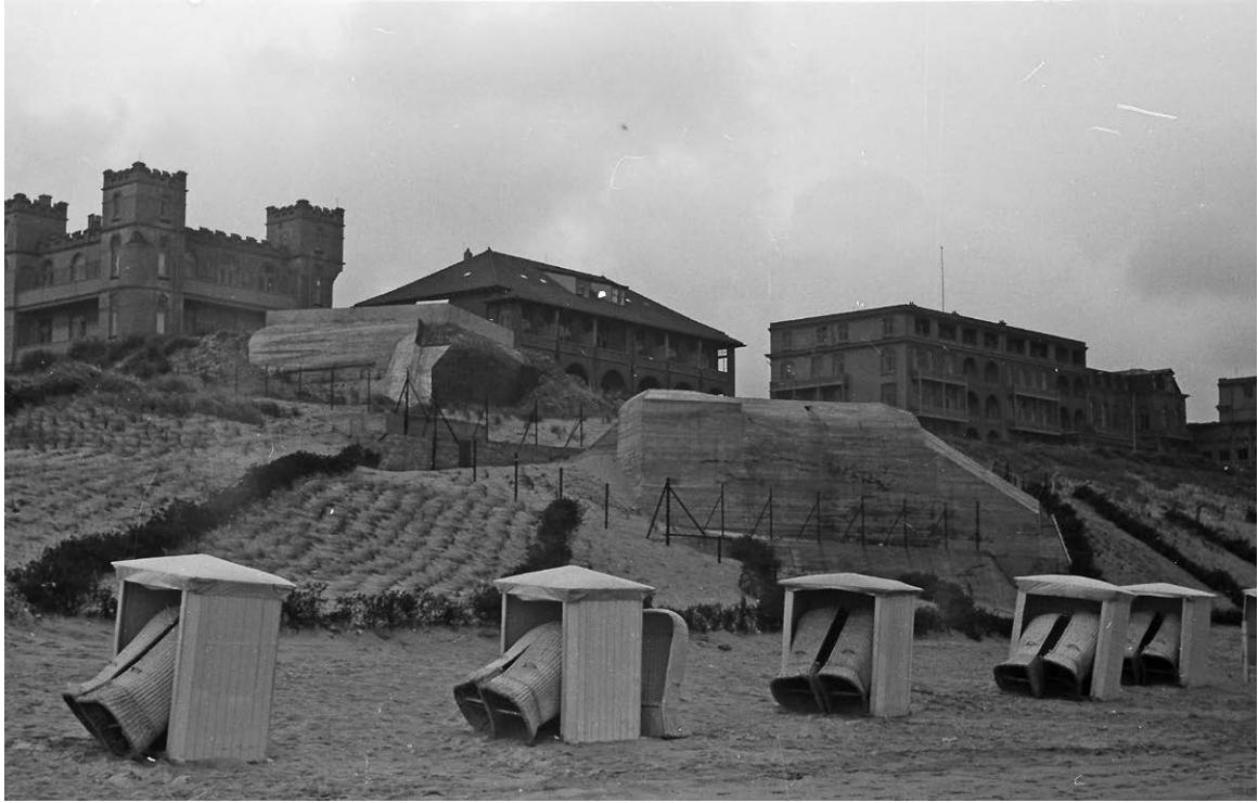
Fig. 4 German gun bunker in front of the Huis ten Duin hotel, Noordwijk, 1947
