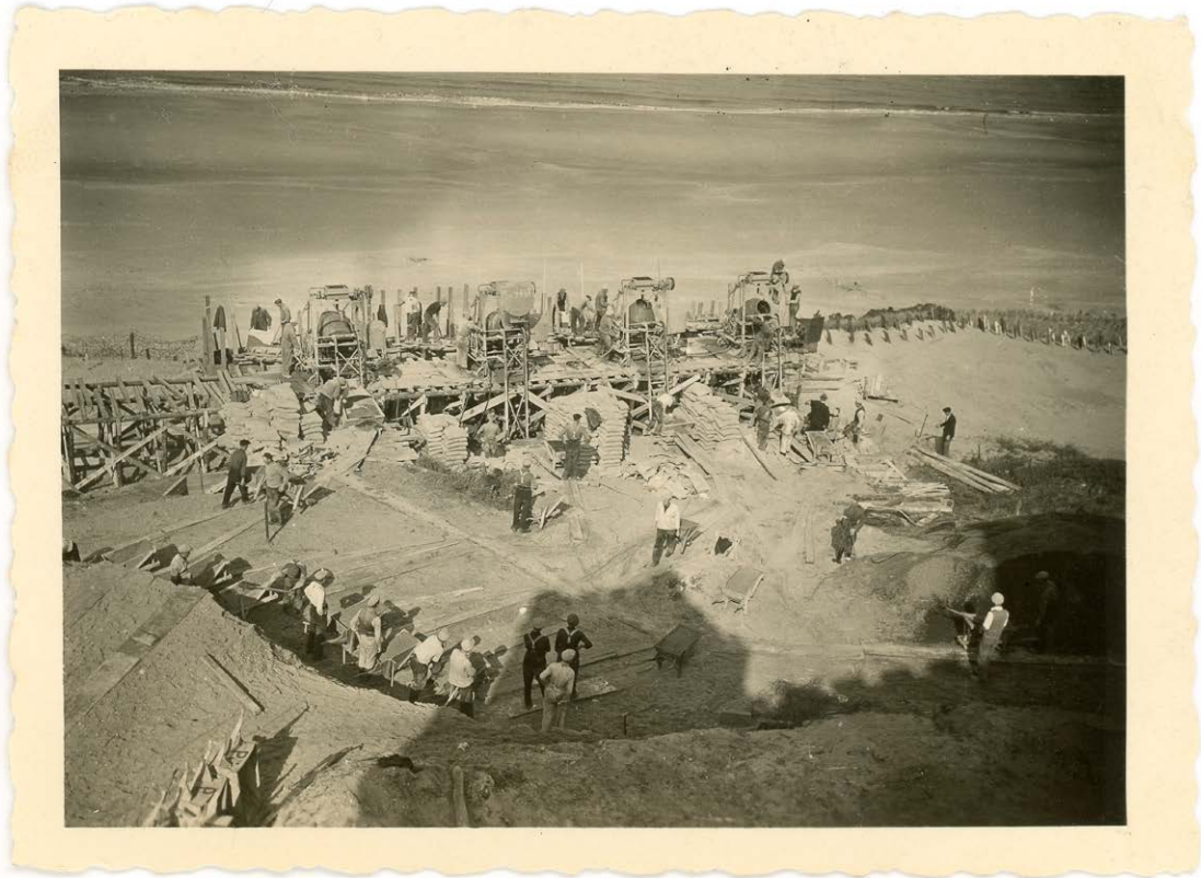
Fig. 27 Construction of a tank wall near Katwijk
