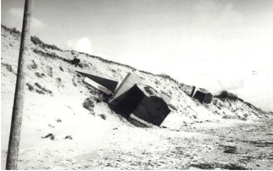
Fig. 18 A bunker collapsed and fell on the beach at Voornes Duin 1966
