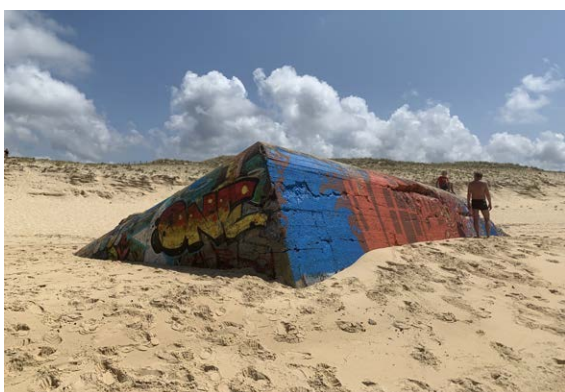
Fig. 28 Bunker located on the beach due to coastal erosion in Contis (France)
