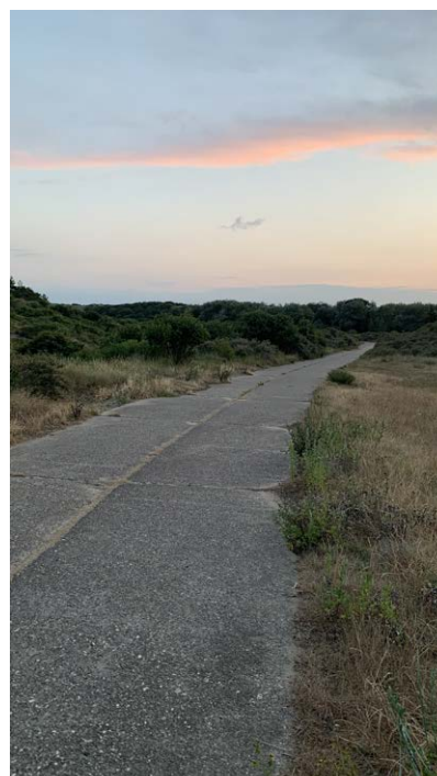
Fig. 31 A road built by the German occupiers in the Festung IJmuiden, also an example of a 'soft trace' of the Atlantikwall
