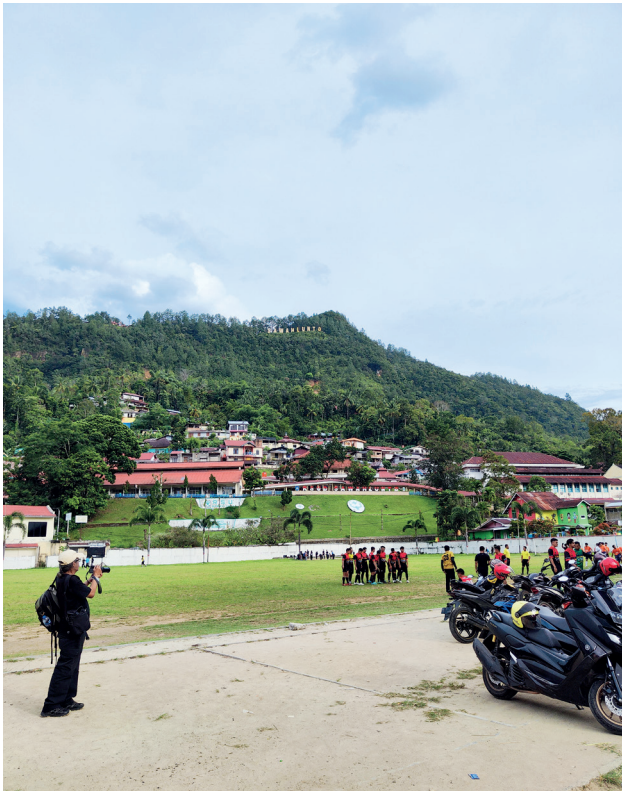
Left: View of the Sawahlunto Hospital - Located behind the community sports field. The limited land in Sawahlunto led to the hospital being built on a hillside with a small area of land
