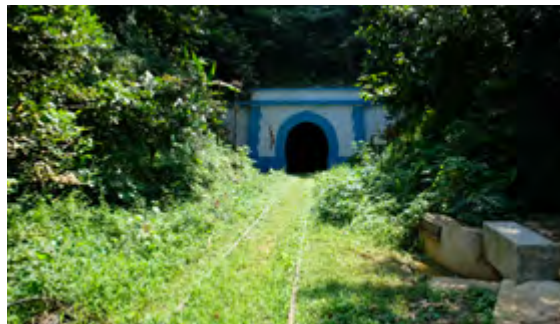
Kalam railway tunnel in 2019
