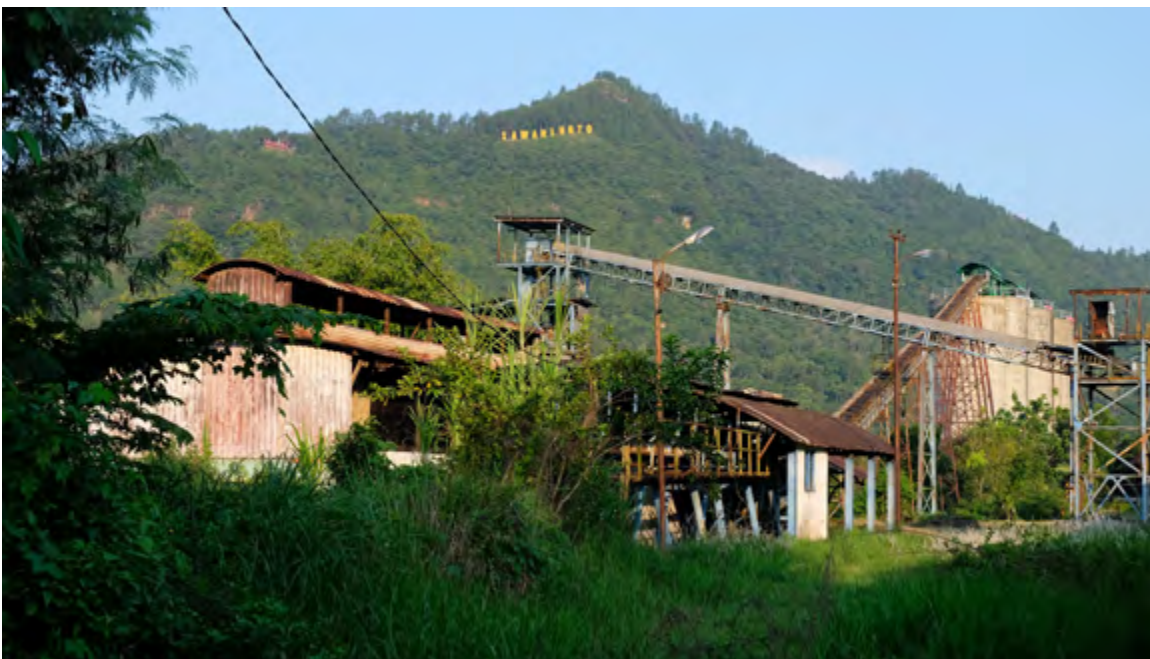
Coal Processing Plant Compound (Area Saringan)
