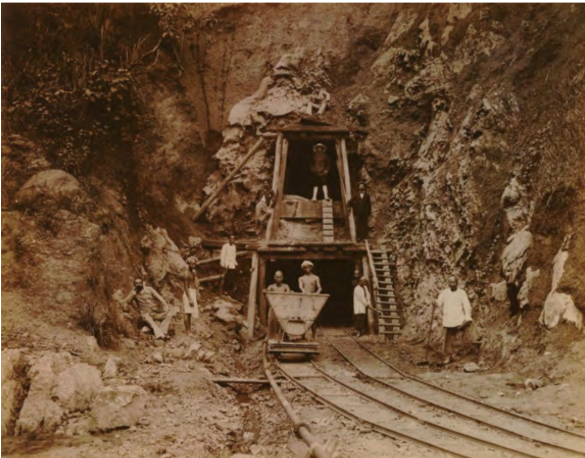
Kalam railway tunnel, as part of the Padang-Sawahlunto track, at the time of its construction (KITLV Collections)
