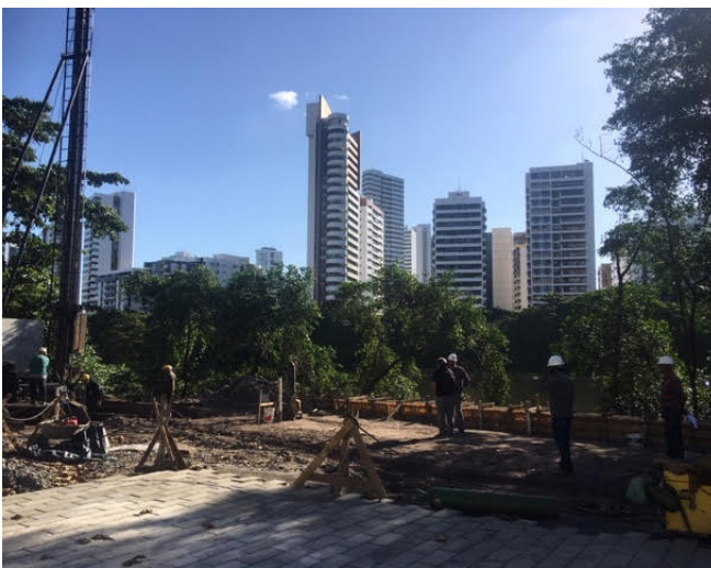
Construction taking place in the Graças neighbourhood (photo: Luiz Vieira).
