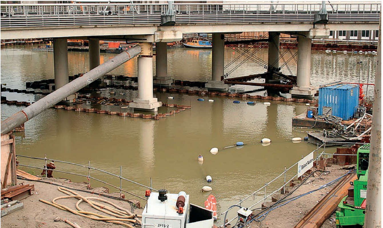
Figure 47. Flooded street during construction work.
