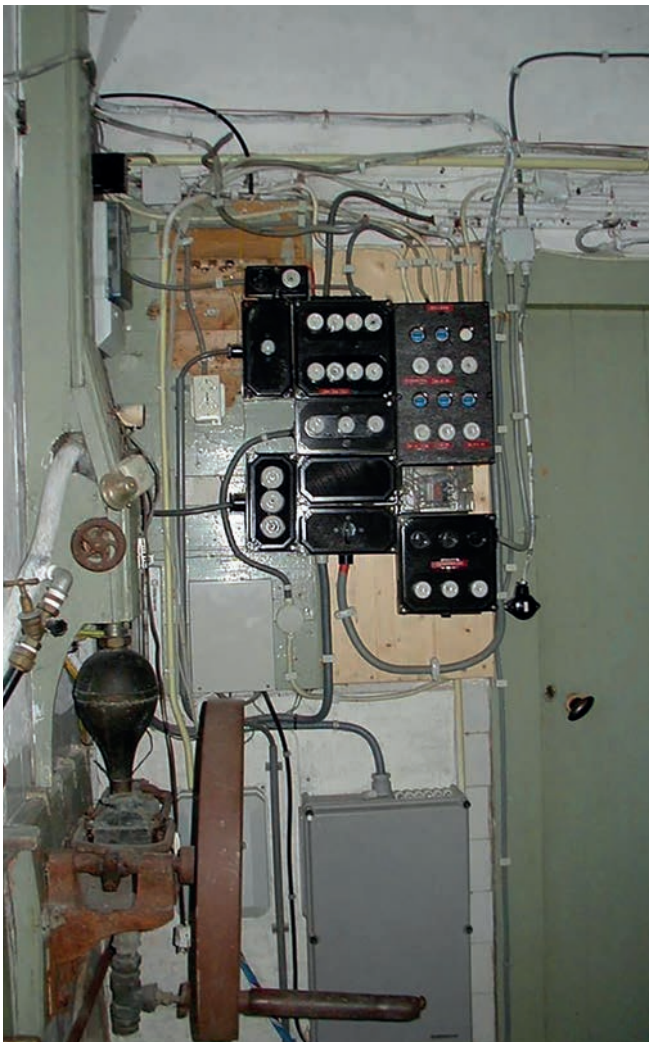
Figure 57. Fuse boxes: an electrical source of fires
