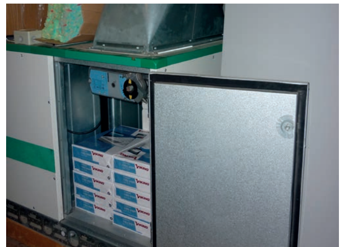
Figure 2. Assessment of the climate control system at the Martena Museum revealed that it did not reduce climatic risks to the collection; the plant has been shut down and serves now as storage for supplies.
