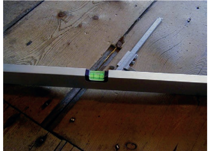
Figure 32. Worn down floorboards at the top of the stairs where visitors turn a corner
