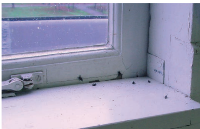
Figure 81. One of the best places to find intruders such as flies, mosquitos and wasps is the windowsill
