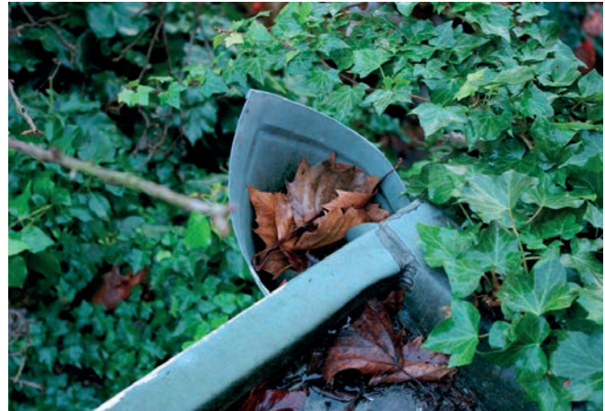
Figure 53. Inspection reveals that leaves clog the rainwater downpipes
