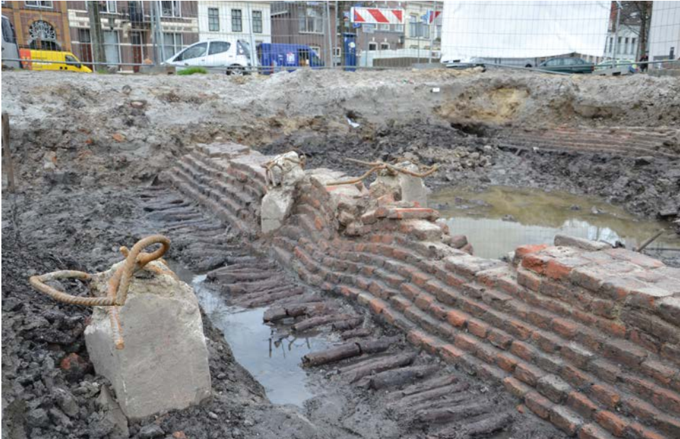
Figure 6 Foundations of a medieval hospital complex (Geertruidengasthuis, Kampen), only slightly disturbed by piles.
