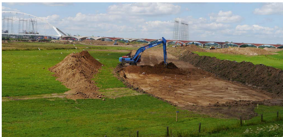
Figure 2 Excavation work in Nijmegen prior to the construction of a side channel of the Waal river (photo: www.ruimtevoordewaal.nl ).
