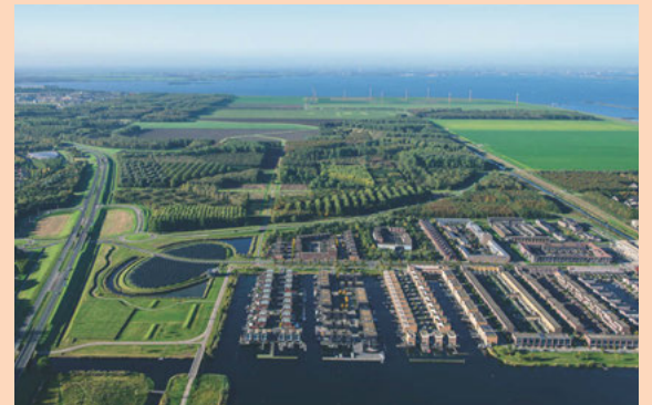
An example of this approach is Zoneiland (Sun Island) near the Noorderplassen-West housing development, Almere. Water heated up by the island's solar panels is pumped into the municipal district heating system.
