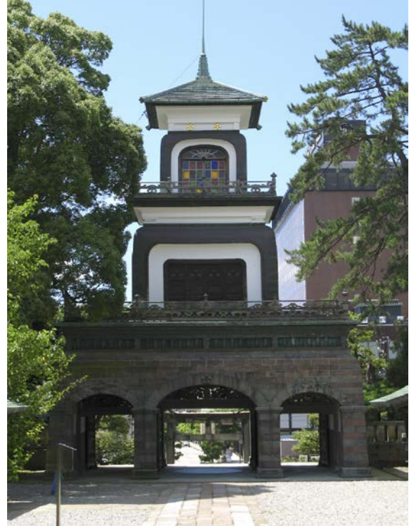
Figure 52 The Oyama shrine gate (Fg2, 2007)
