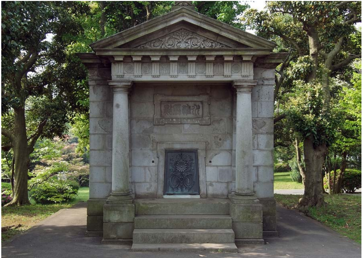
Figure 49 The Japan Standard building in Tokyo (Wiiii, n. d.)
