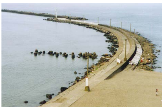
Figure 51 The Escher embankment (柵の香り, n.d.)
