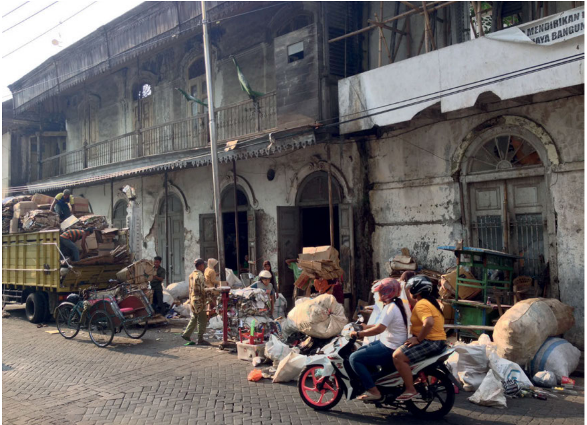
Dilapidated buildings in Indonesian inner cities point out the necessity of revitalization.
