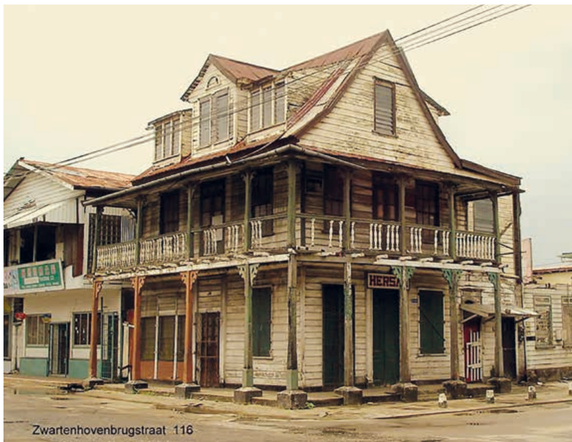
Photo 7: Dilapidated building historic inner city Paramaribo.
