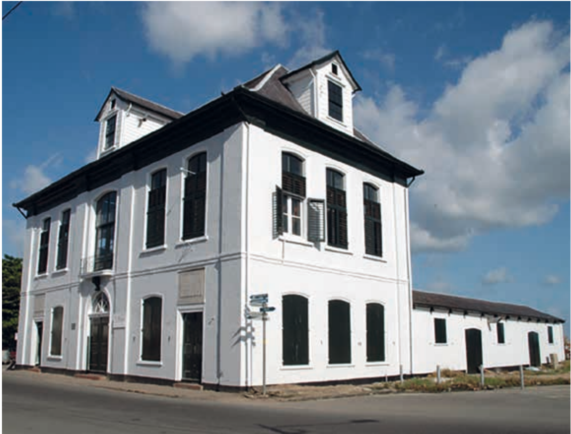
Photo 10: Restored building De Waag in Paramaribo.
