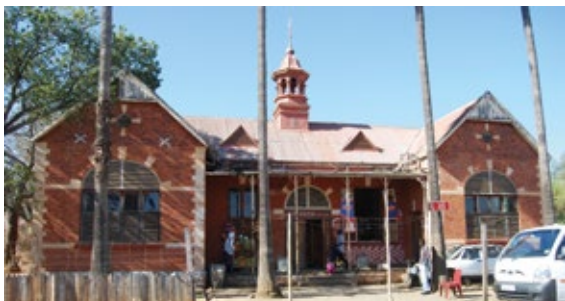
Old Administration building
