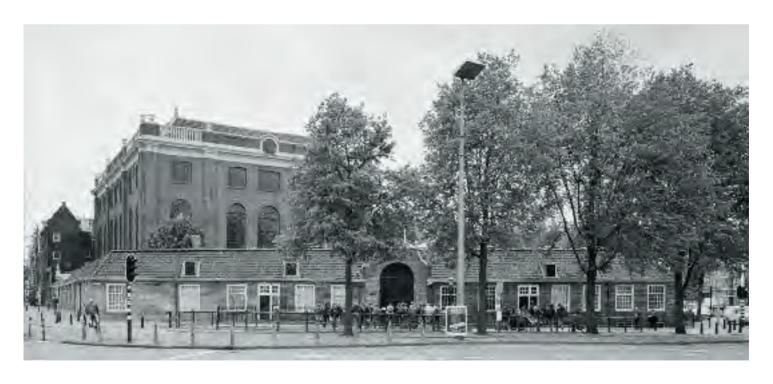
103 The west wall of the annexes. This photograph clearly shows that the placement of the windows in the section at the Muiderstraat corner (on the left) was altered during the restoration in 1954-1959.
