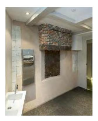
108 The floor of the basement was lowered. It was originally just below the seventeenth-century iron hearth-plate and white tiles (witjes) on the wall.
