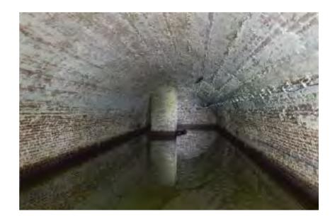
118 The brick barrel vaults under the Snoge. The imprints of the centrings are clearly visible.
