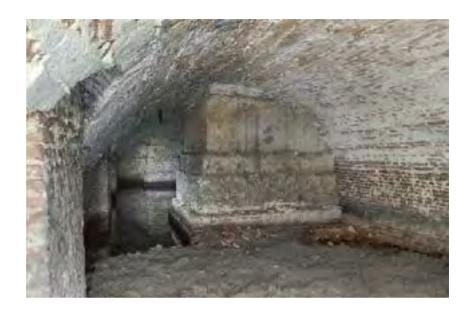
117 The brick barrel vaults under the Snoge and the masonry foot of the column passing through the vault.
