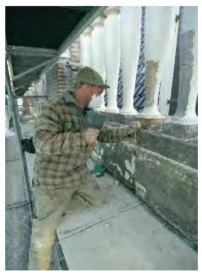
121 Raking out joints and earlier repairs to the sandstone parts of the balustrade.
