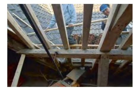
120 Re-laying the Snoge's roof tiles The date 28 September 1788 is visible on the purlin.
