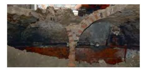
stumbled upon an underground cistern beneath the entrance gate. The existence of this cistern was unknown to us during the planning stage. It was not possible to adapt the plan for the new cellar and leave this cistern in place (fig. 126).
