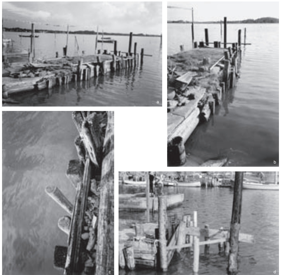
Fig. 34 Schleswig: photographs of dam from fig. 33.
